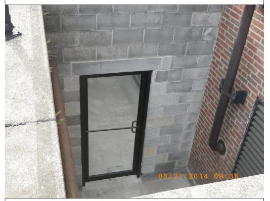
Solution to eliminate the fall hazard and use of a wooden pallet as a ladder. A door was installed within the block wall to allow access to area two from area one using the roll up garage door. The new door also closes automatically to still create the function of a baffle for the air intakes. One Water Front loading dock trash compactor
