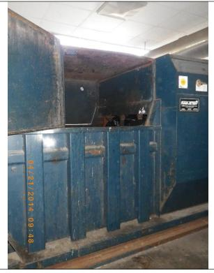
Trash compactor located on loading dock. Trash bags need to be lifted above recommended safe height and placed into the compactor. This would be very hard for employees that are not very tall or strong.
