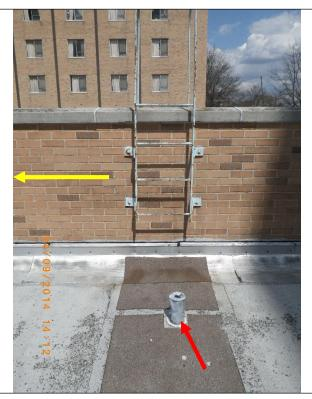
View from upper roof looking towards the ladder. Vent pipe (red) appears far from this angle, but as photted above is close to the exiting motion from the ladder. Solution was to move the ladder approximately 10' left (yellow) and reinstalled, where no hazards where presents.
