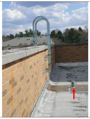
Access ladder on towers roof from upper roof to lower roof located over the ERC café. A vent pipe (red) was located near the bottom of the ladder is posed a potential trip hazard when exiting the ladder.
