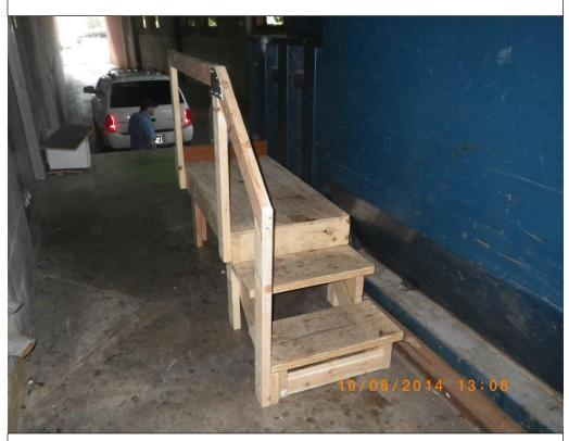
Solution to eliminate a possible back strain/sprain or other injury. A platform was constructed and installed to allow the trash to be placed into the compactor at a more reasonable height.
