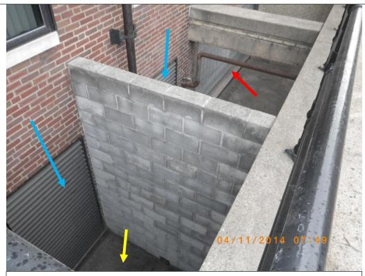
Concrete block wall which separates the pit into two areas. The block wall is necessary and designed to baffle the pit for adjacent air handling unit intakes (blue). Area one is located upper right (red) with access from the roll up door. Area two is located lower left (yellow) and accessed by pallet.
