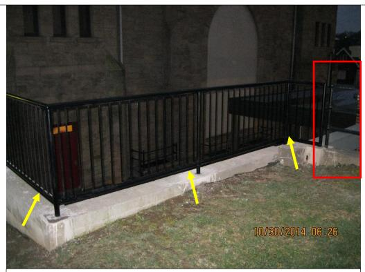
No railing was previously present. A 12' fall hazard to the lower road was present. A matching hand rail set to industry standards of 42" was constructed and installed. The old three post rail can be seen in the upper right (red). The new hand rail (yellow).
