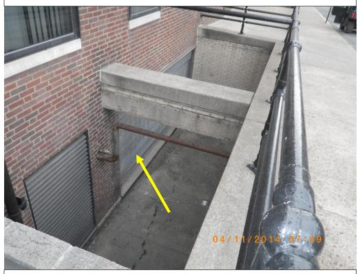
The pit was divided into two areas, separated by a concrete block wall. The one area of the pit could be accessed from within the building using a roll up garage door for entry (yellow).
